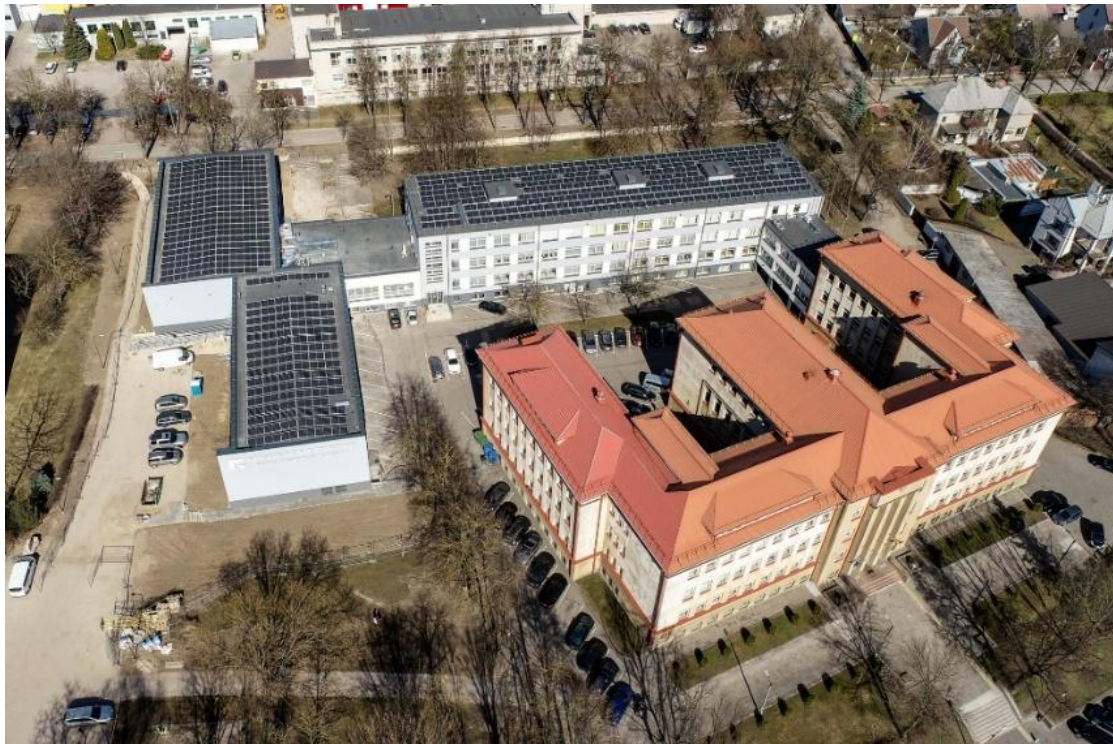
Fig. 2. Panel installation on the roof of Lietuvos Inžinerijos Kolegija Higher Education Institution Source: created by authors
