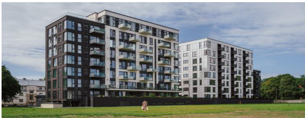
Fig.3 Residential building Toom-Kuninga 21, Tallin,Estonia
